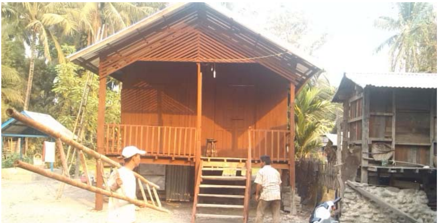
Work is being performed on one of the churches.
